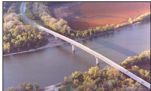
The Shippingsport Bridge, a vital link between two Illinois communities, was expected to take three years to replace. The new bridge shown here was completed in only two years.
