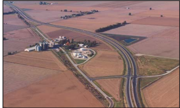
The IL-29 Expressway, shown here as it bypasses Berry, IL, features innovative drainage solutions uncommon for rural highway designs.
