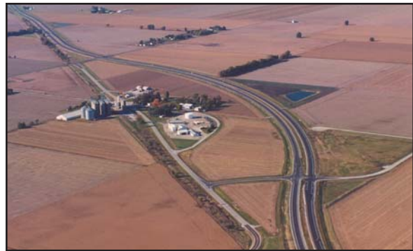
The IL-29 Expressway, shown here as it bypasses Berry, IL, features innovative drainage solutions uncommon for rural highway designs.
