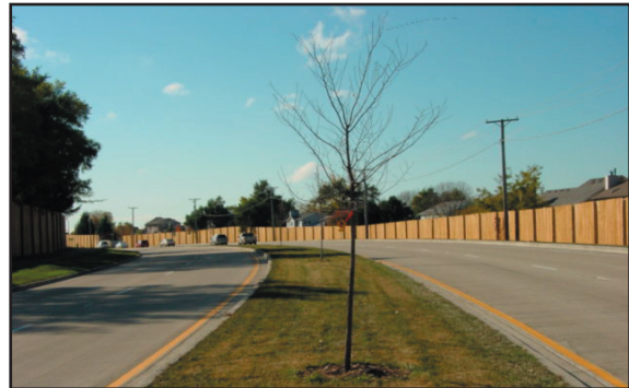
The landscaped 16 ft. raised median on Orchard Road is a context sensitive solution that brings an aesthetic appeal to the new roadway.
