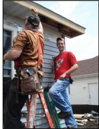
Chris Stritzel, senior engineer, stands with nail gun at the ready as another volunteer lines up a piece of the soffit.
