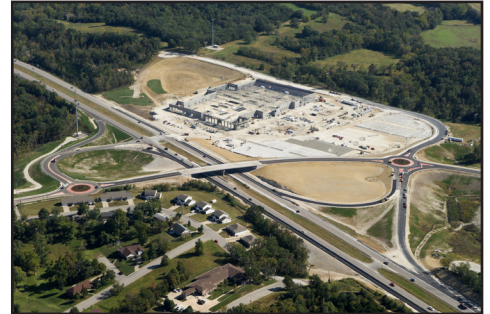
The U.S. 50/City View Drive Interchange is the first known 2-Quadrant Type-A Parclo Interchange with Roundabouts in the U.S.
