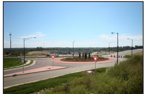
The use of roundabouts was among the Practical Design elements that contributed to a combined project savings of $1.4 million.
