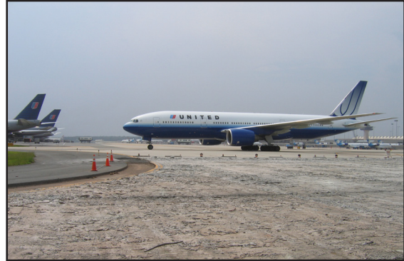
Maintaining operations at this major international airport was a critical factor in project phasing.
