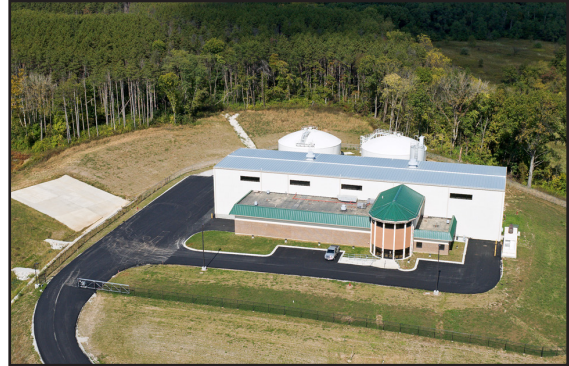
The treatment plant is designed with the flexibility to operate with either sand or membrane treatment.
