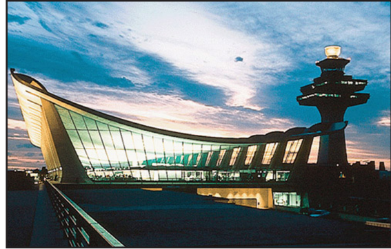
CMT has been working at Dulles International Airport since 1982.
